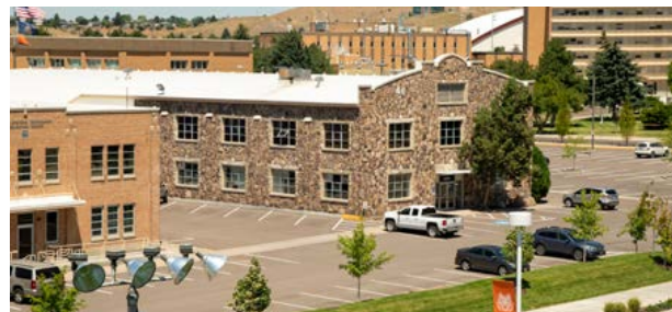
ESTEC + Vocational Arts Existing Conditions
